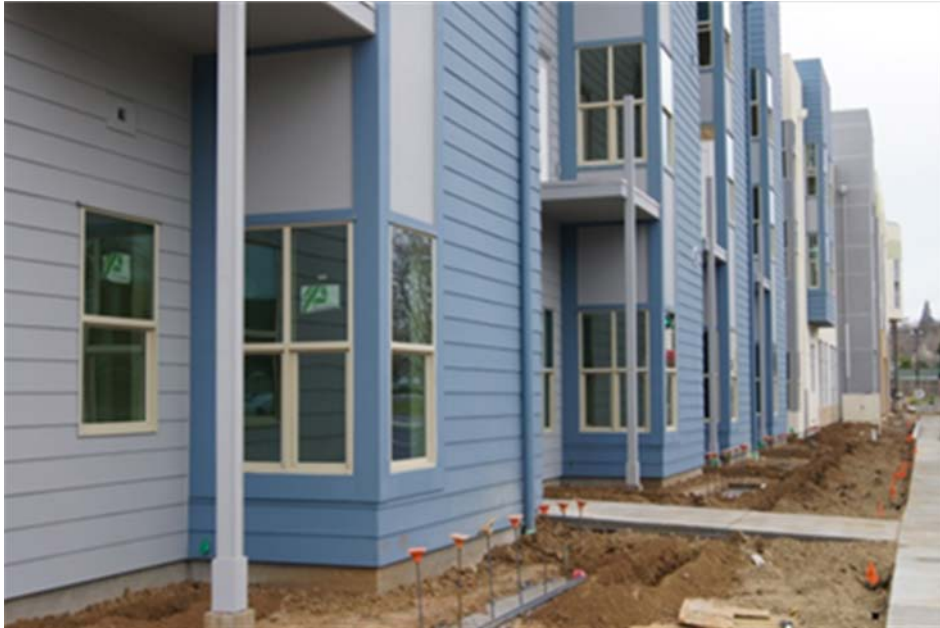
Figure 15: Low-Rise Multifamily in Final Phases of Construction
