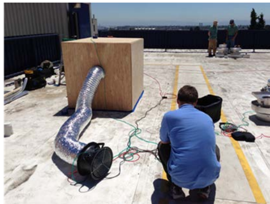
Figure 10: Rooftop Exhaust Fan Flow Capture Hood and Duct Blaster
