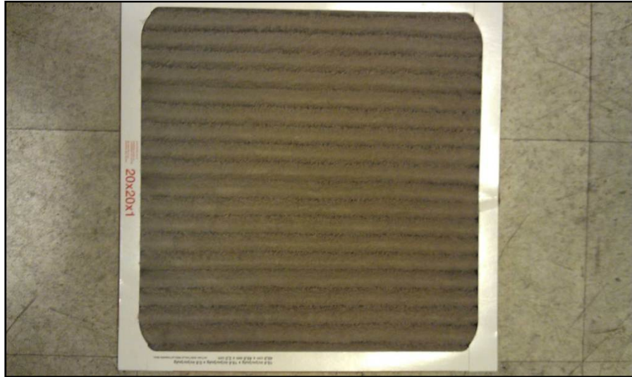
Figure 40: Original Filter Installed in the Hallway of House 5
