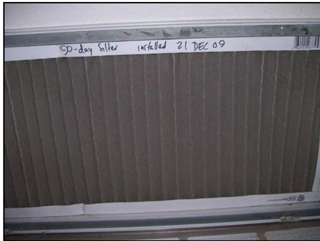
Figure 12: House 2 Initial Filter that was Very Dirty at the Start of Data Collection
