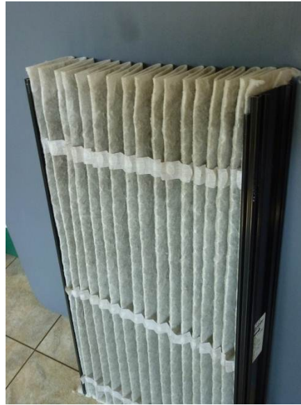
Figure 87: Original 4 in. Deep Pleated Filter Installed in House 10 at the Start of the Study
