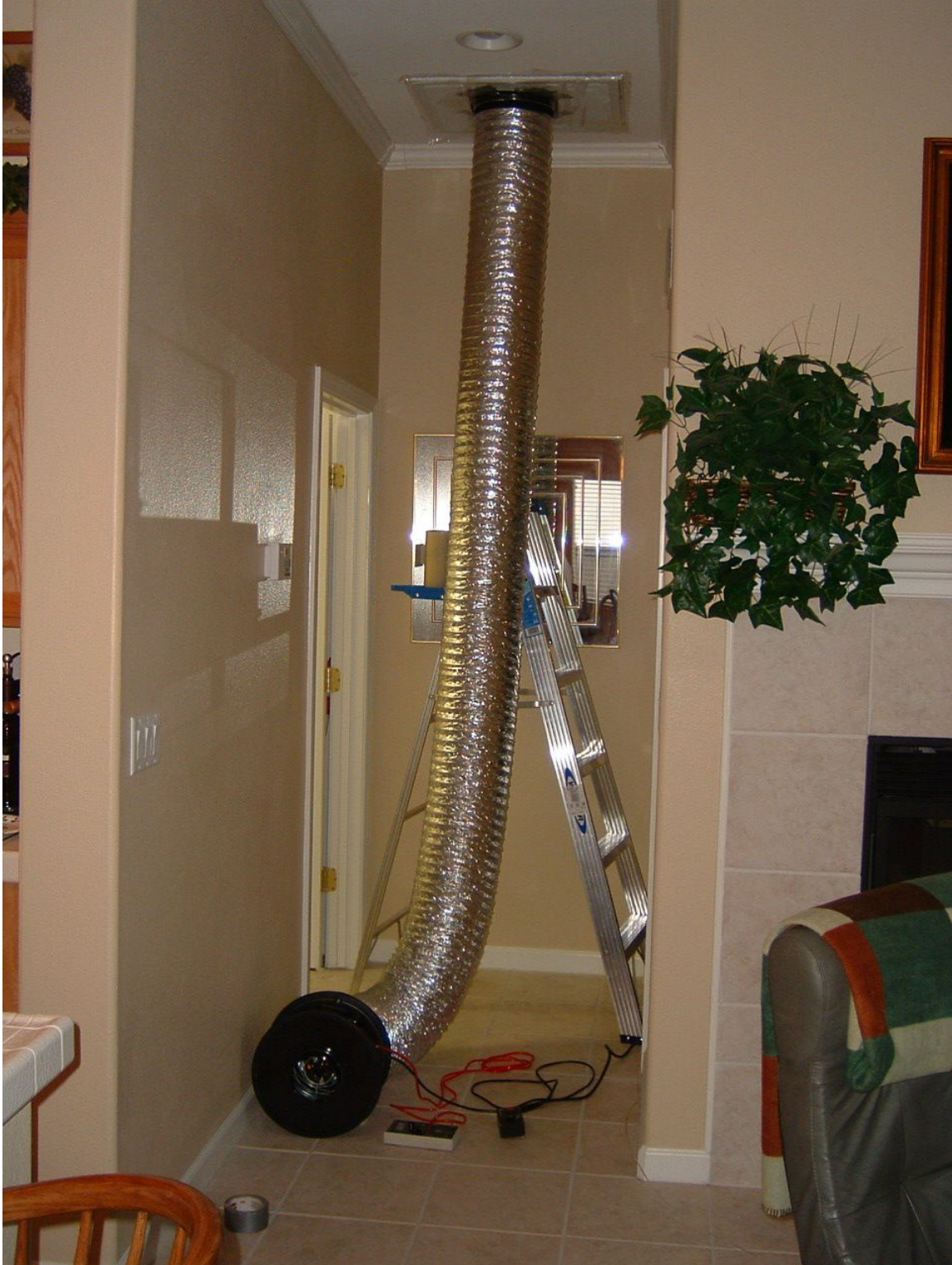
Figure 4. Pilot Home P2, Duct Blaster installed at return air inlet of forced air heating/cooling system.
