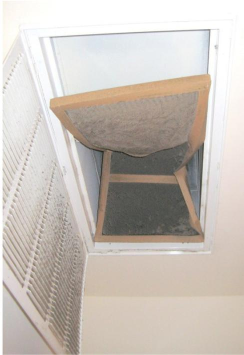
This 14 in. X 30 in. X 1 in. standard filter is so dirty it is sucked into the return duct that is substantially smaller than the return grille. The home owner is sufficiently embarrassed that he offers to go to the store and bring back a new filter. He is instructed specifically to bring back a low efficiency, low cost filter.
