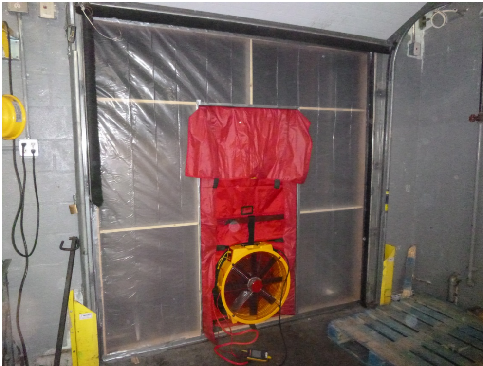
Figure 2: Dock door air leakage test apparatus
