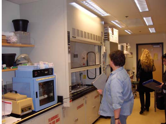
PES Demo hood prior to retrofit
