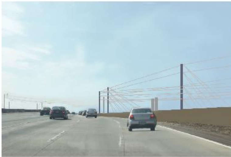
Simulated with project view looking southbound on I-5, north of the proposed transmission structure associated with the proposed Units 8 and 9 line of units depicting the revised design of the proposed transmission system.
