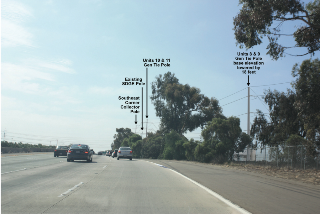
Simulated with-project view looking southbound on I-5, north of the proposed transmission structure associated with the proposed Units 8 and 9 transformers depicting the revised design of the project transmission system.
