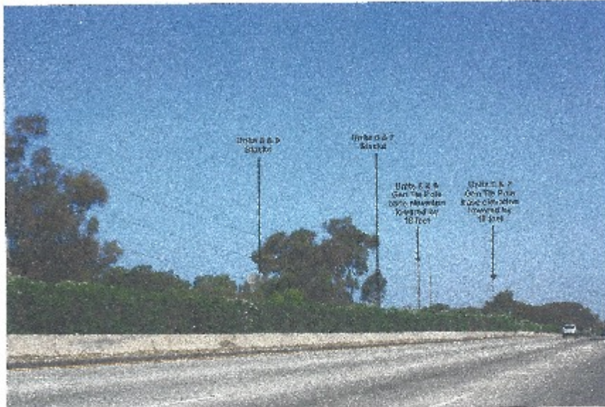
Similar to the subject view looking northbound on I-5 south of the proposed transmission structure associated with the proposed Units 8 and 9 transformers depicting a revised design of the project transmission system.
