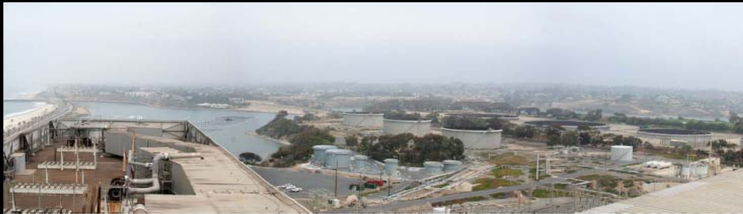
1. Panorama from top of turbine building looking north
