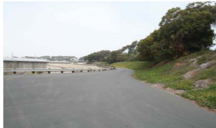
3. Internal road on project site looking northwest
