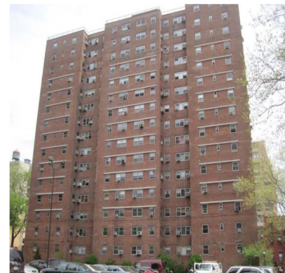
3. Post-War two-pipe steam
