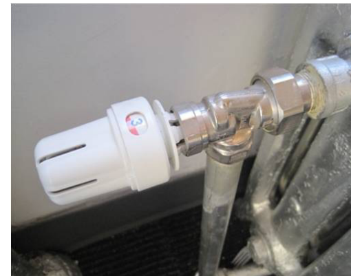
Thermostatic Radiator Valve (TRV)
