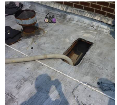
Cavity between roof deck and top floor ceiling
