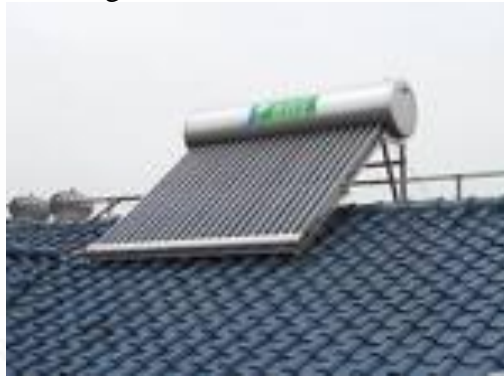
Figure 15: Solar water heater
