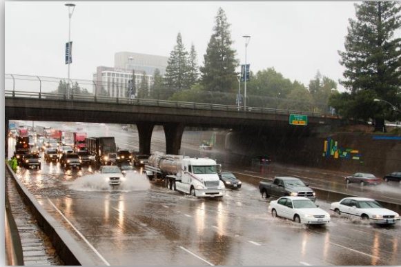
I-5, Sacramento, Oct. 13, 2009 Photo: California Department of Transportation
