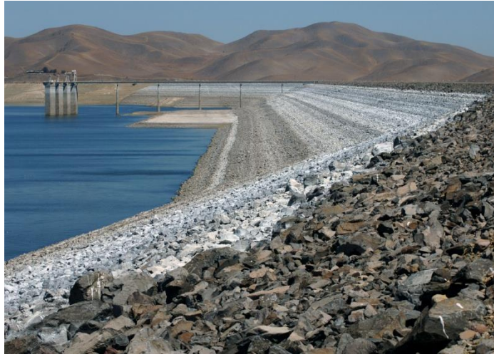
California Department of Water Resources San Luis Reservoir; July 11, 2007
