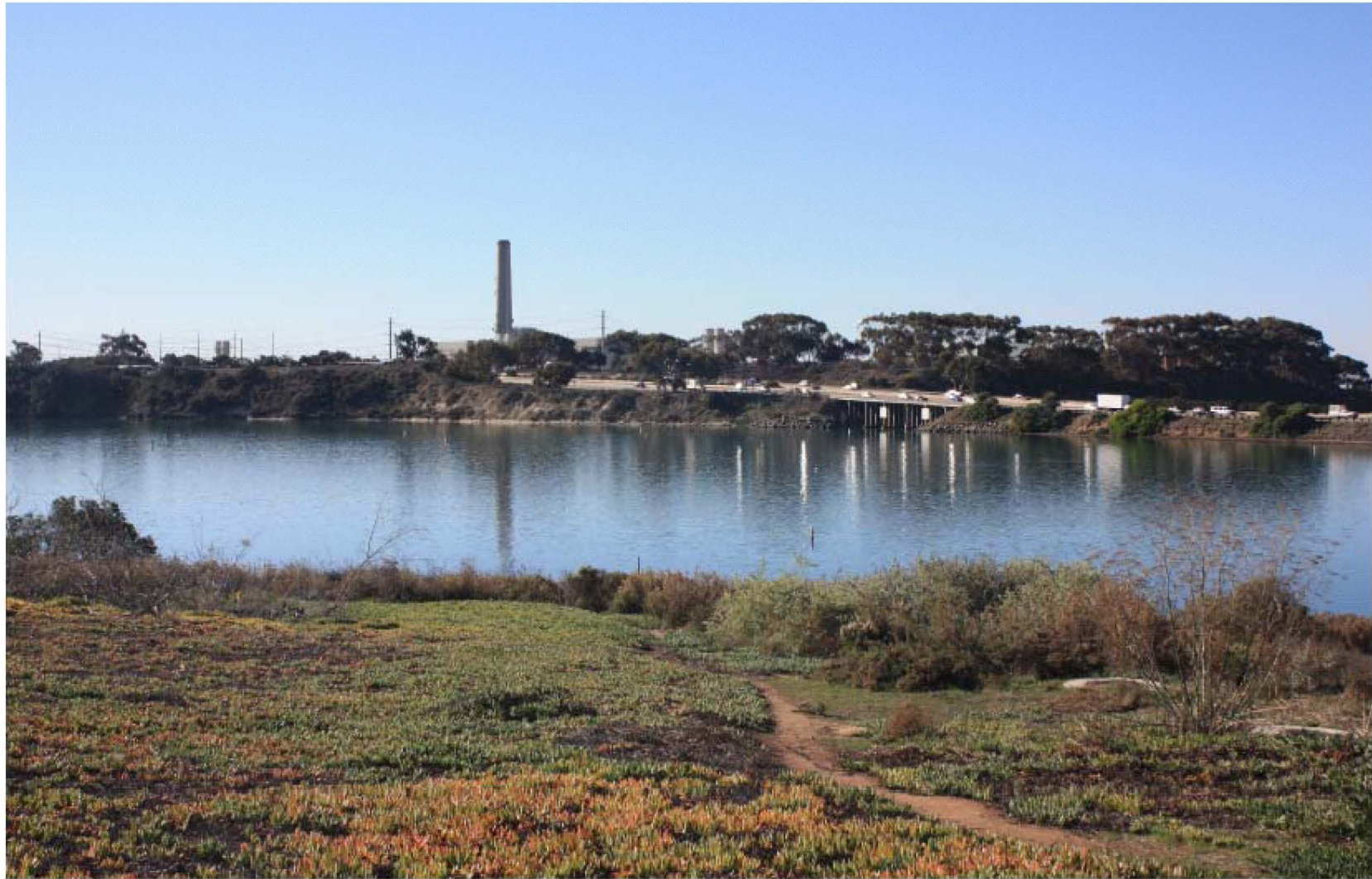
View from the end of Hoover Street toward the project site with the Amended Project power generation and transmission facilities in place, before removal of the Encina Power Station.
