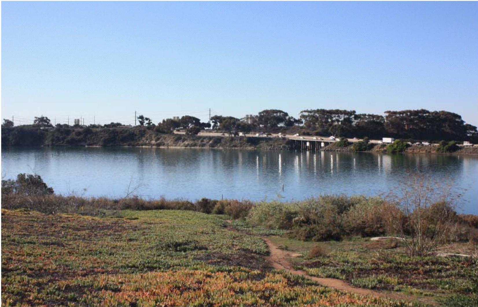
View from the end of Hoover Street toward the project site with the Amended Project in place, including removal of the Encina Power Station.
