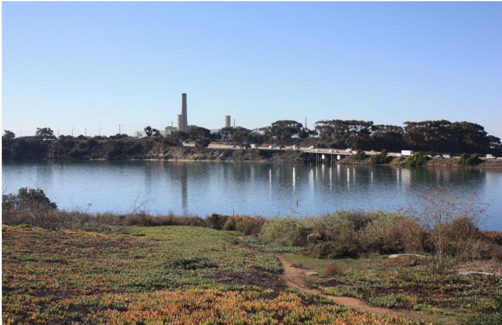
Baseline view from the end of Hoover Street toward the project site with the licensed CECP in place.
