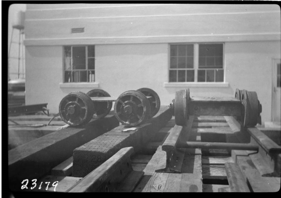
Barre Substation control house, September 27, 1940; Copyright: Southern California Edison Photographs and Negatives collection of The Huntington Library (Call No. 2-23179 / Image No. SCE_2_23179).
