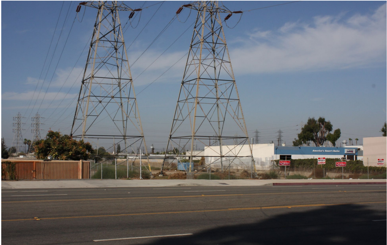
G. Katella Avenue looking north Views toward the project site are screened by intervening structures and vegetation.
