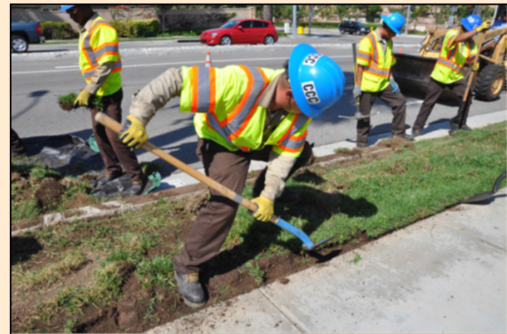
CCC removing turf in the City of Corona
