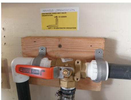
A greywater diverter valve and examples of greywater irrigated garden beds
