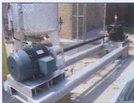
Figure 1: Typical Fan Drive Arrangement
