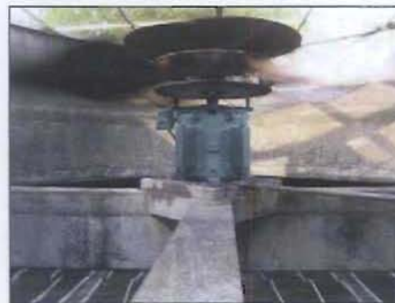
Figure 7 – PM Motor Installed in Place of Gearbox & Driveshaft
