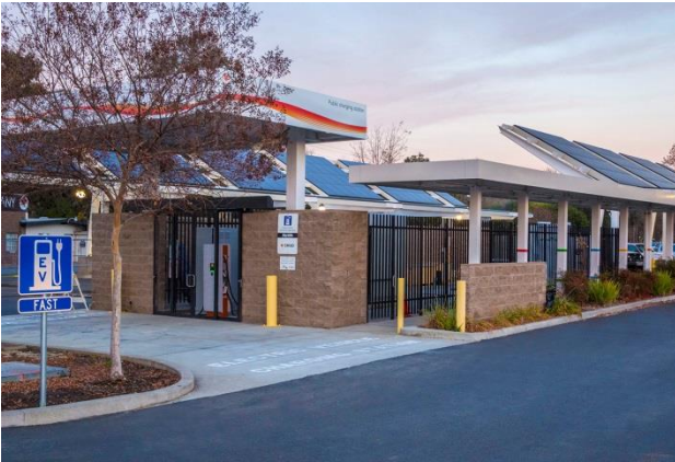
SMUD Headquarter Operational Since March 2014
