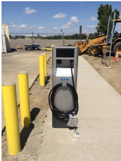
Airport Under Construction Cell Phone Lot (4/14/16)
