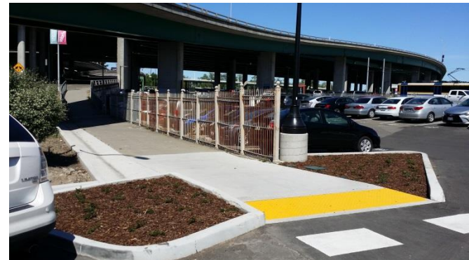
Amtrak Sac Valley Station Site Pre Construction
