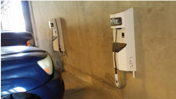
Sac Food Coop Level 2's Installed
