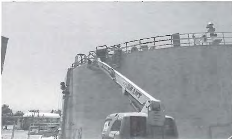
RP-2 Digester 4 Improvements
