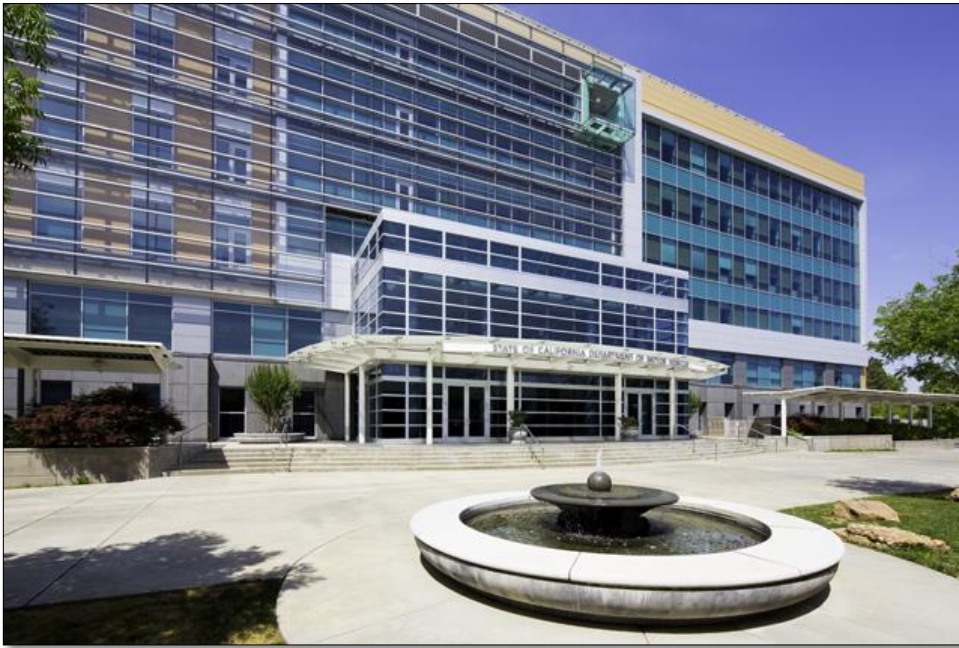
Photo. DMV Headquarters, Sacramento, LEED Silver Renovation, CVAIA Award Winner. Source: California Department of General Services
