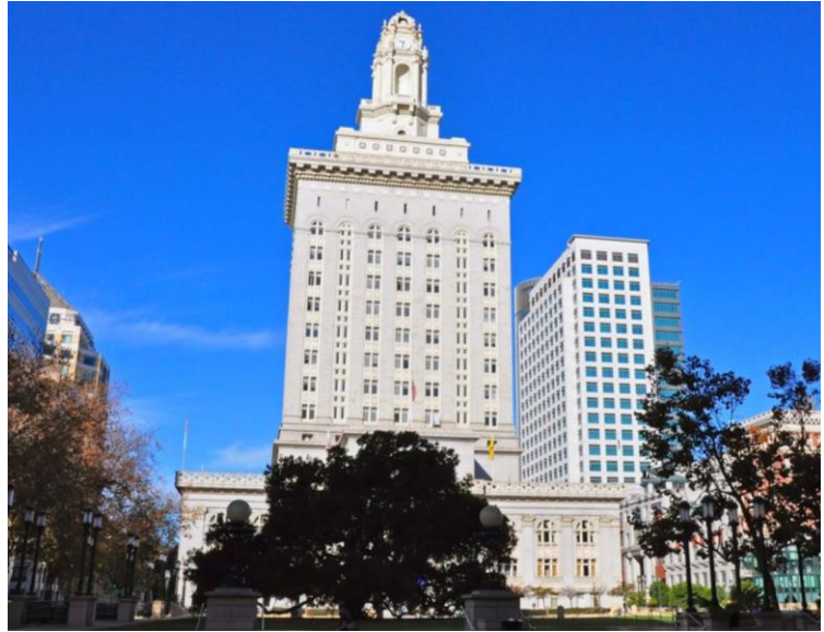
Oakland City Hall Energy Efficiency Upgrade Photo by Yuri Krasov
