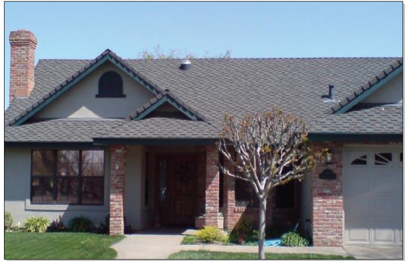
Photo: Grupe Homes, 2009, Energy Star with Home Performance Retrofit
