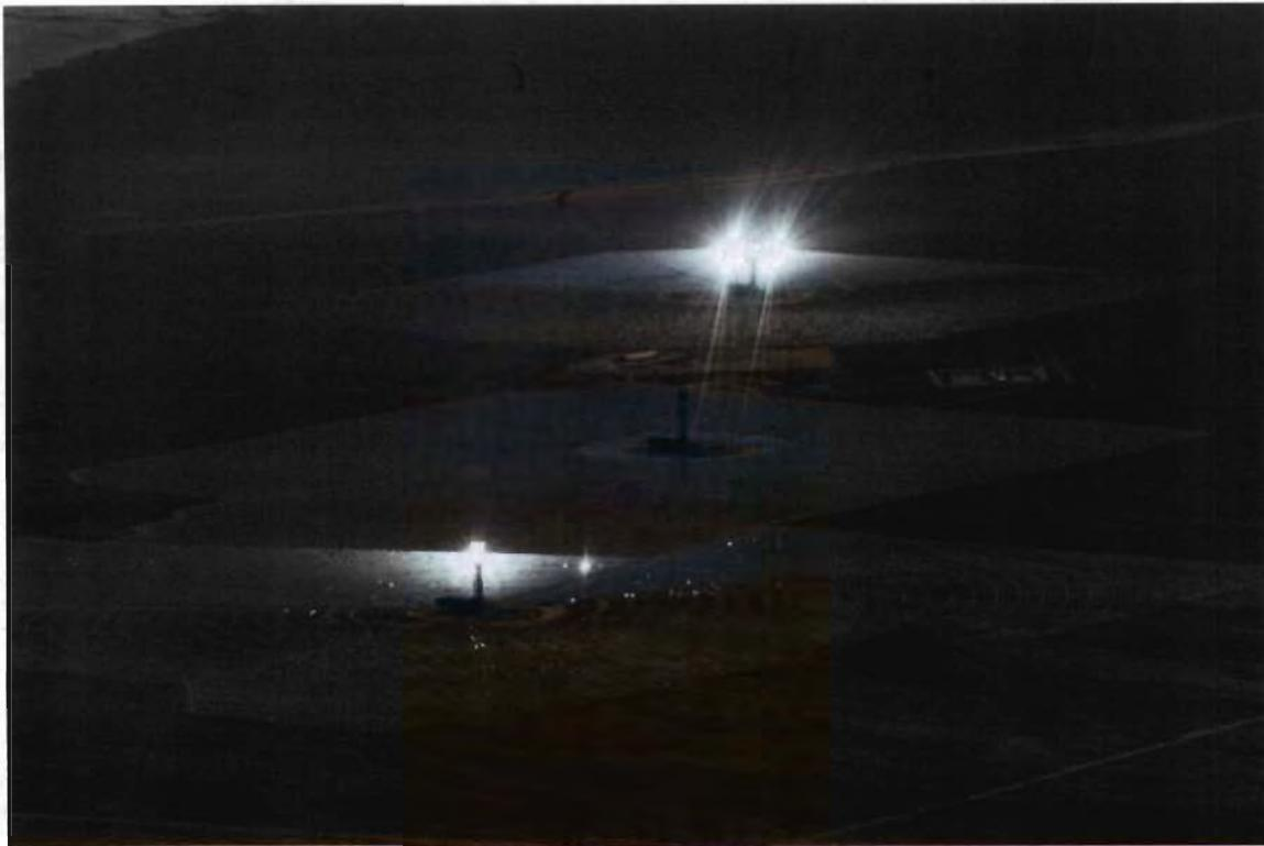
**Photo 2.** *Photo of the ISEGS site taken from the north. From left to right: Tower 1; Tower 2, not in operation; and Tower 3. The photographer's position in relation to heliostat position and orientation results in no DSRH from Tower 1, but strong DSRH from Tower 3 which causes disability glare.*
