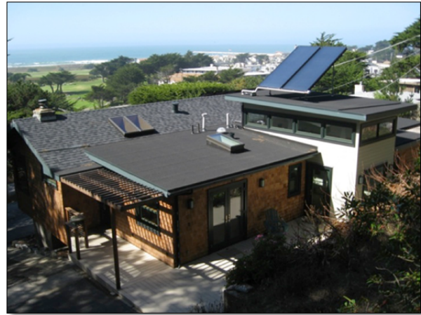
Photo. Deep Retrofit of California Beach Home, Source: Lawrence Berkeley Labs, Environmental Energy Technologies Division eetd.lbl.gov
