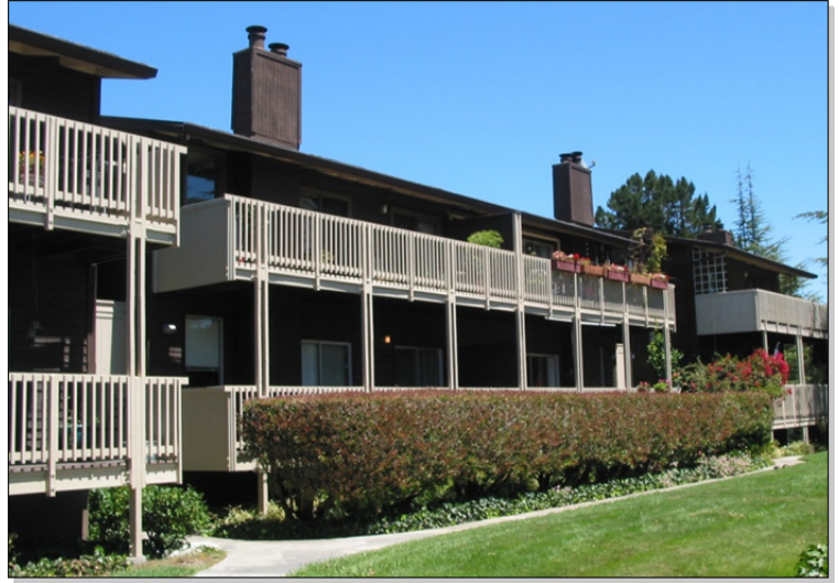
Photo: W. Charles Perry, Lauriedale Apartments San Mateo, CA, Comprehensive Energy Efficiency Assessment, 2007.
