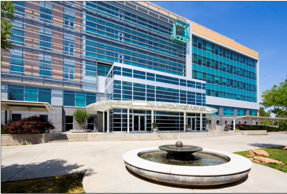
Photo. DMV Headquarters, Sacramento, , LEED Silver Renovation, CVAIA Award Winner. Source: California Department of General Services
