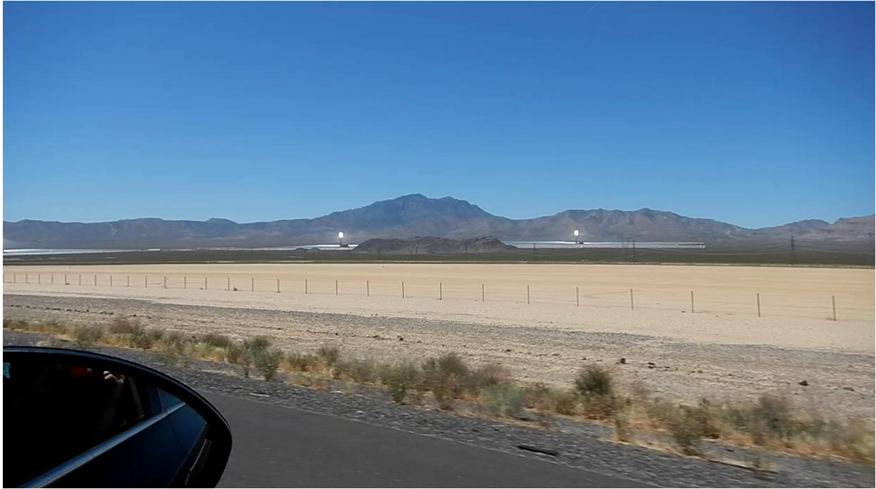
Figure 12. Photograph of illuminated receivers at Units 2 and 3 while heading southbound along I-15.
