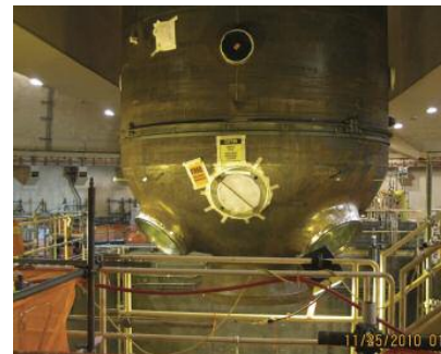
The RSG is lifted onto a purpose-build platform, skidded into the building, and then set into its final position by the containment vessel's internal crane
