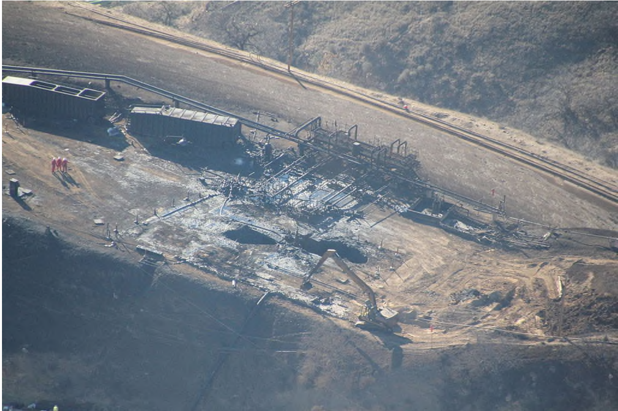
Leak site. Image: Earthworks
