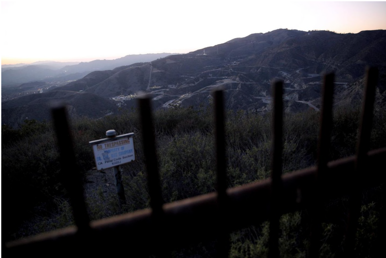
A "No Trespassing" sign and fence mark the boundary of the SoCalGas Aliso Canyon Storage Facility, looking toward where a leaking gas well and a relief well are being
