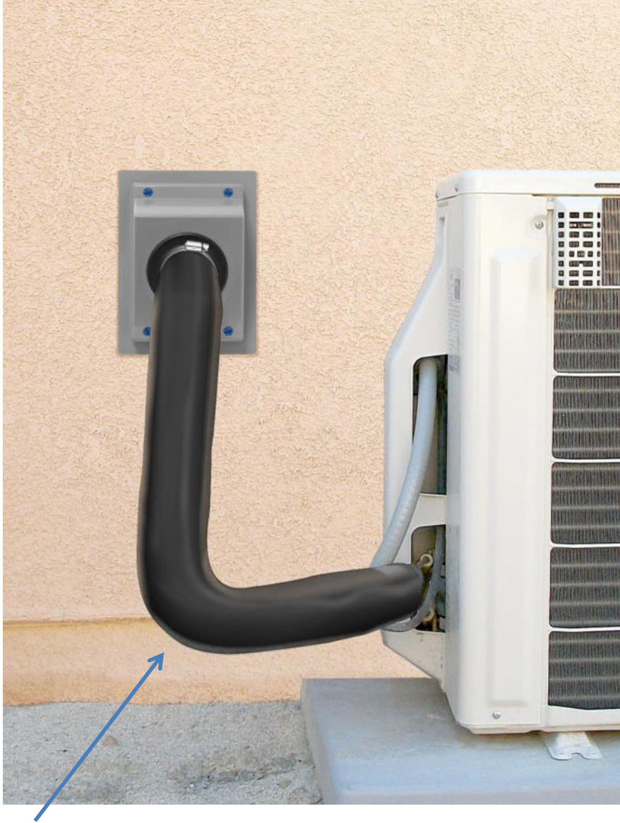
Vapor retarder & insulation protection
