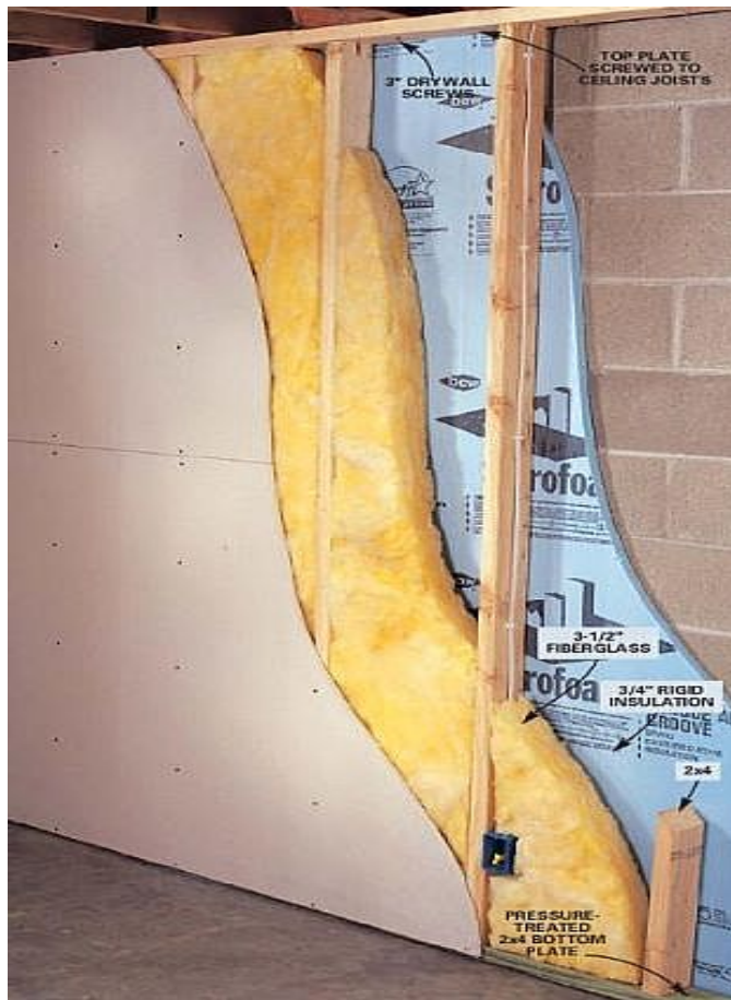
Figure 3-2324 – Masonry Brick Masonry Brick Wall with Furring Details Source: California Energy Commission
