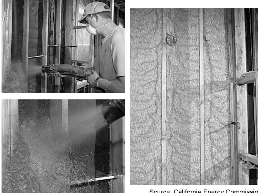
Figure 3-34 – Cellulose Insulated Wall
