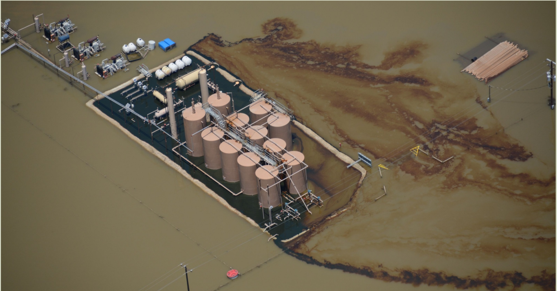
2015 Austin TX Oil and Chemical Plant Failure
