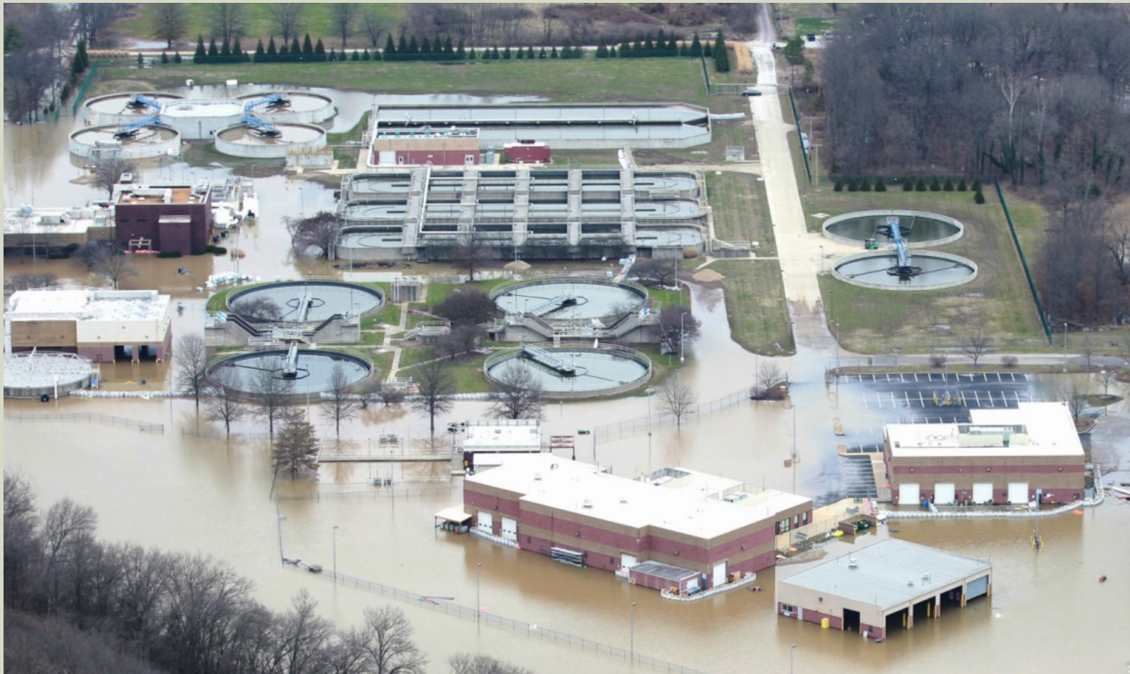
2015 St Louis Sewage Treatment Plant Failure
