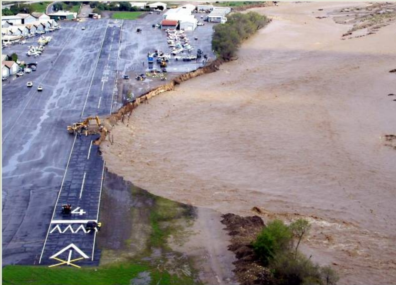
SANTA PAULA AIRPORT FLOOD DAMAGE 2005
