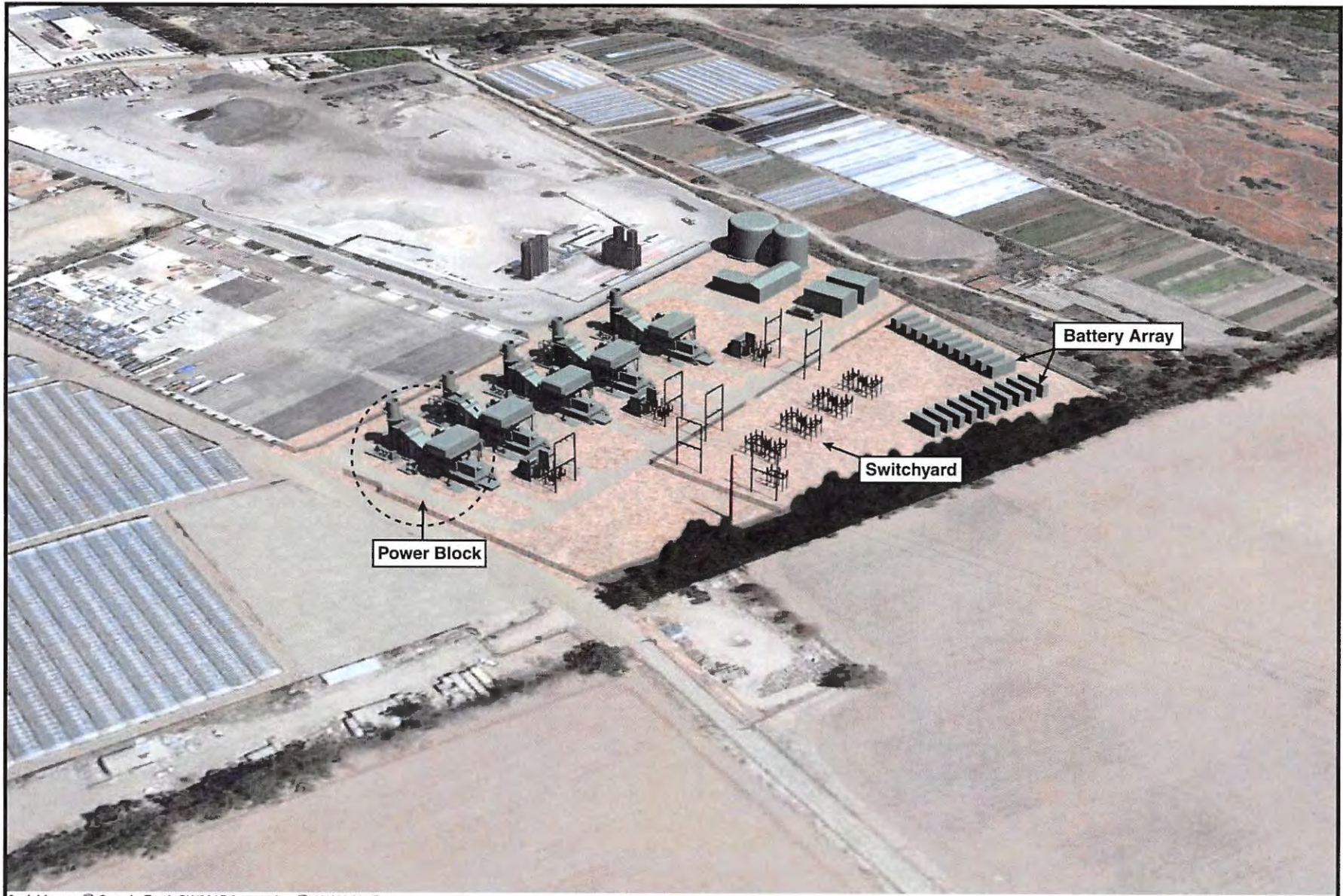
PROJECT DESCRIPTION - FIGURE 2 Mission Rock Energy Center - Architectural Rendering of Power Plant and Battery Array
