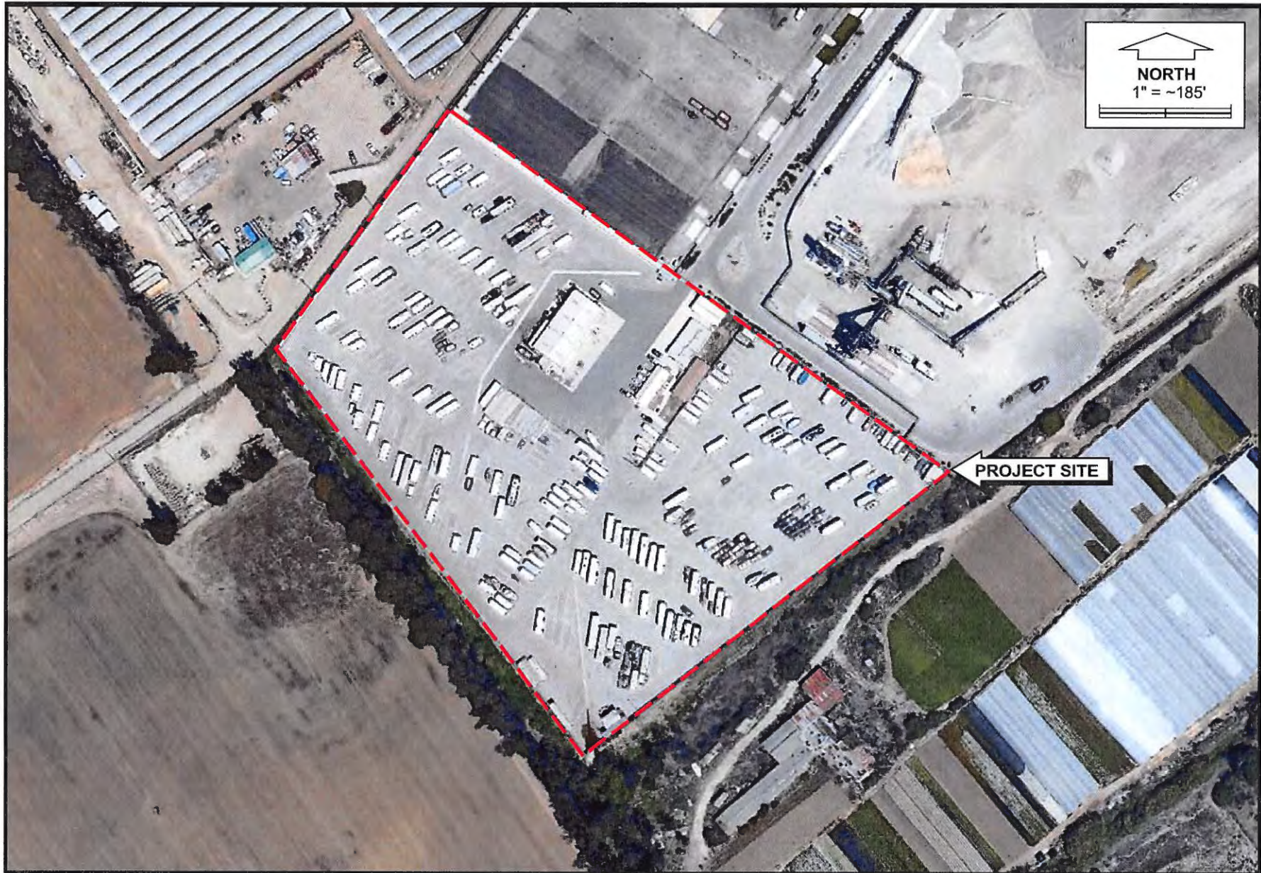
PROJECT DESCRIPTION - FIGURE 5 Mission Rock Energy Center - Project Site - Close up
