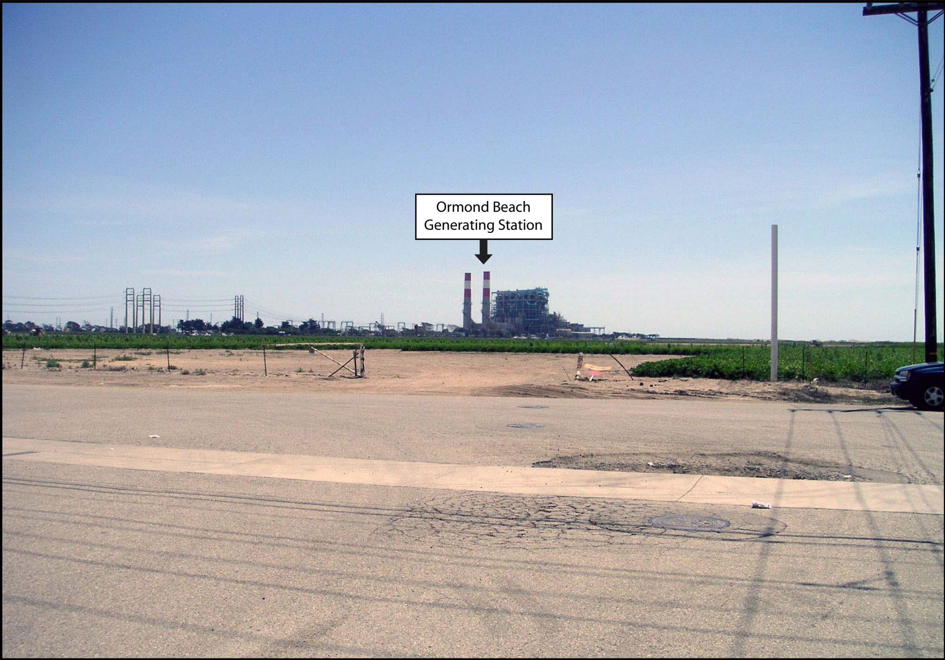
Mission Rock Energy Center - View South toward the Ormond Beach Generating Station from Arcturus Avenue
