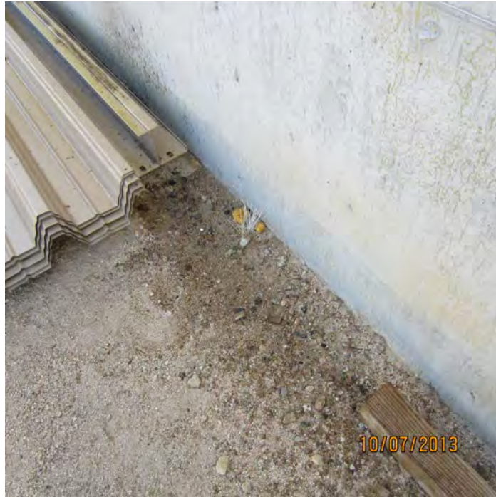
U3 Lube Oil/Mist Eliminator
