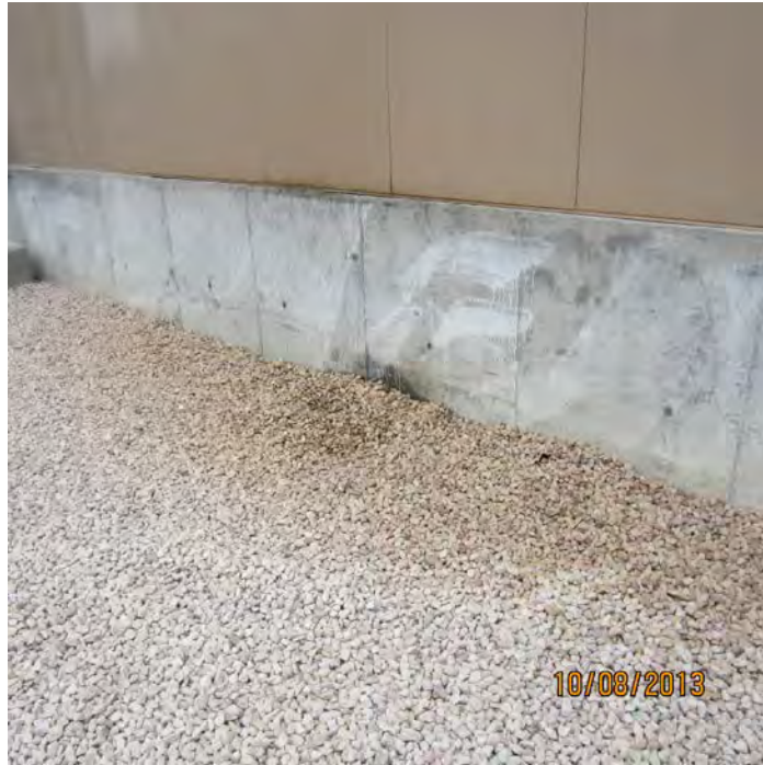
U1 Lube Oil/Eliminator
