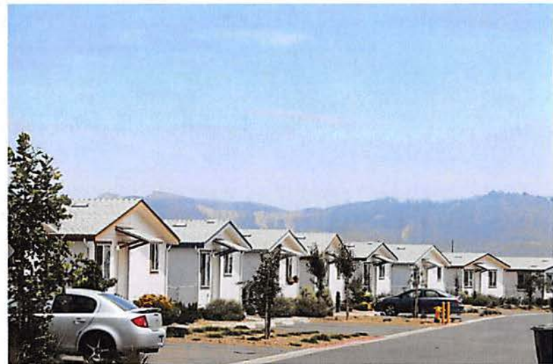
No Updated DPR Form provided for Worker Housing Camp 800
