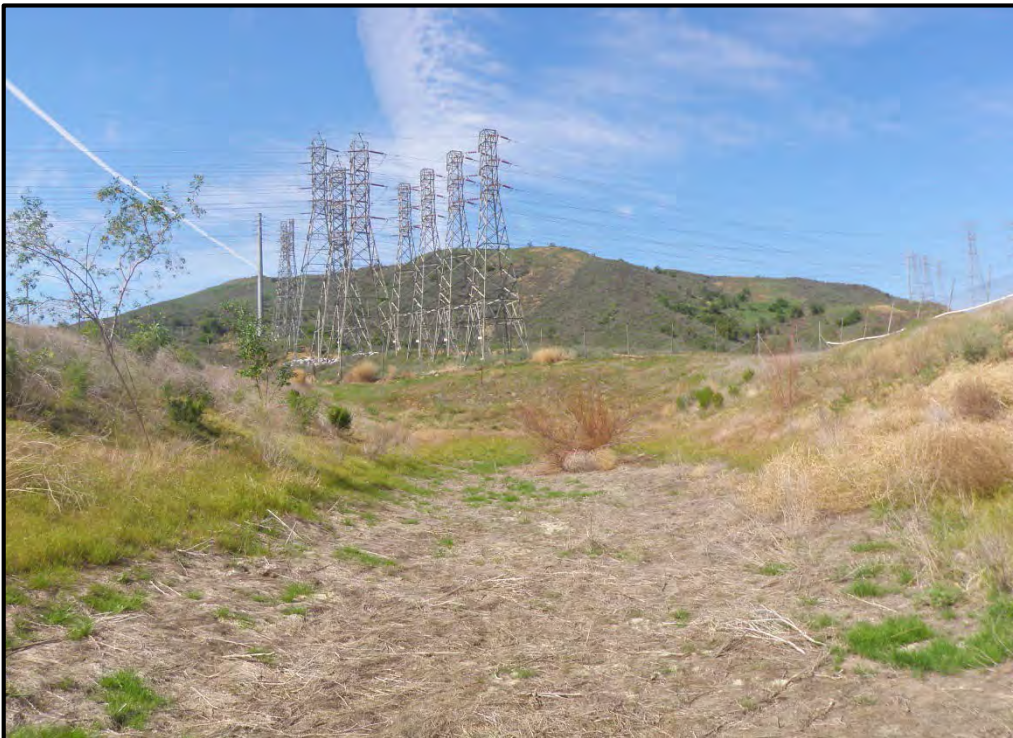
Figure 12. From bottom of pond looking to the northwest towards proposed tower location, March 2, 2016
