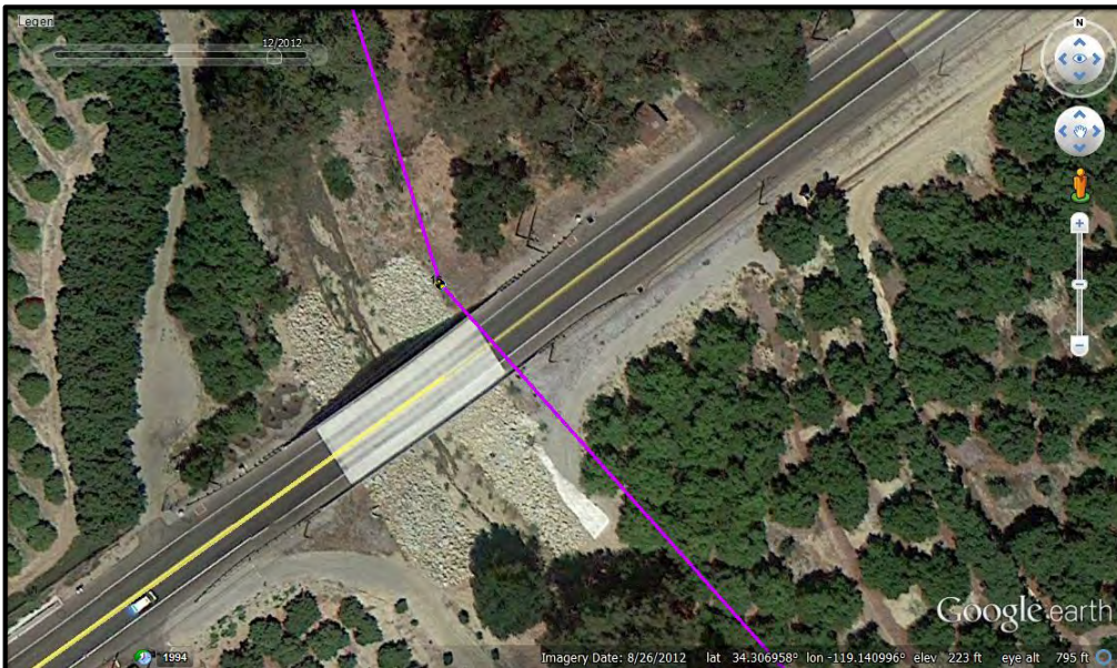
Figure 9. Aerial from August 2012, post vegetation removal and installation of rip-rap along banks.
