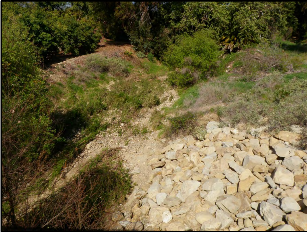
Figure 10. Looking north-northwest from near the proposed tower location at rip-rap and stream channel, active flow channel is approximately 55 feet from the tower location, above the rip-rap embankment.
