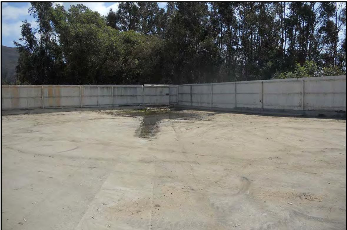
10. Accumulation area of surface water drainage located at the southwestern corner of the Project Site.
