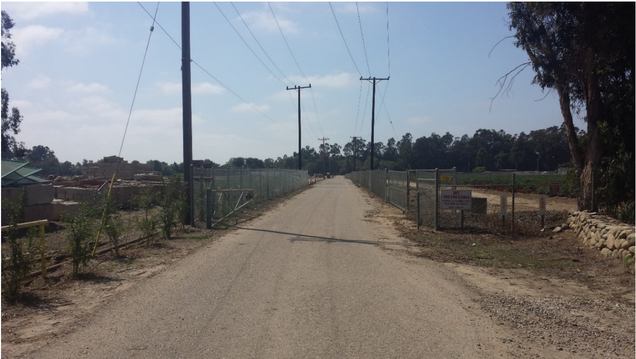
Photo 5. Shell Road, adjacent to the western corner of the Minn-Cal Enterprises RV and Boat Storage yard, facing southwest along proposed natural gas pipeline route. September 22, 2015.
