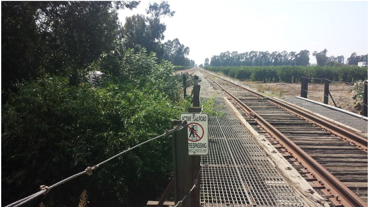
Photo 7. Southern Pacific Railroad right-of-way, at intersection with Todd Road, facing southwest along proposed natural gas pipeline route. September 22, 2015.
