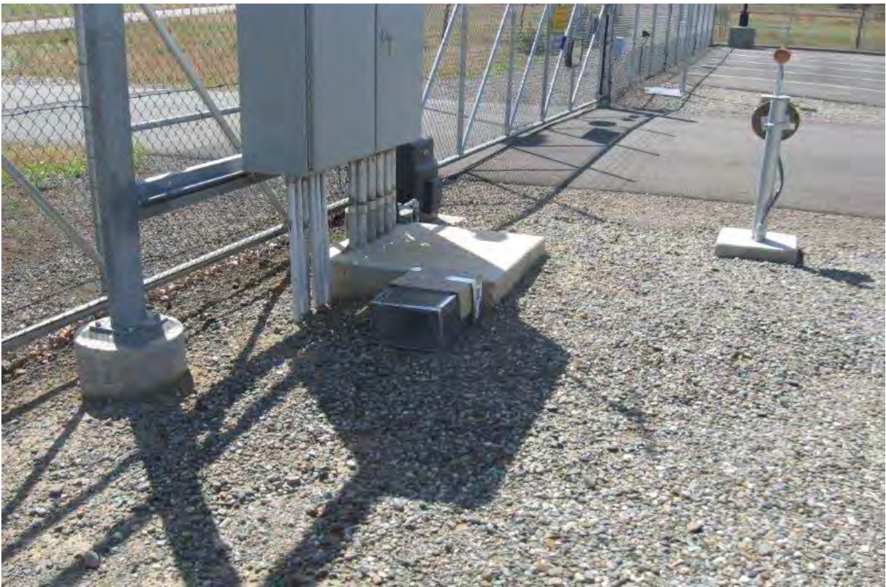
Photo 8, of typical placement of snake traps near plant access points, 4/10/15.
