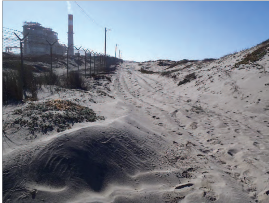
Photograph 5: View of the Access Road. Facing south from the northern end of the Access Road. October 19, 2016.
