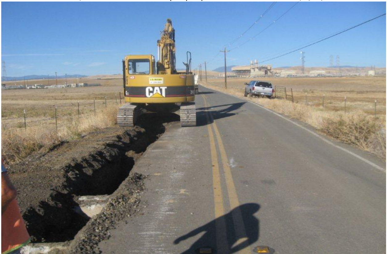
Photo 10, of typical alternate waterline excavation within existing roadway, 10/7/14.
