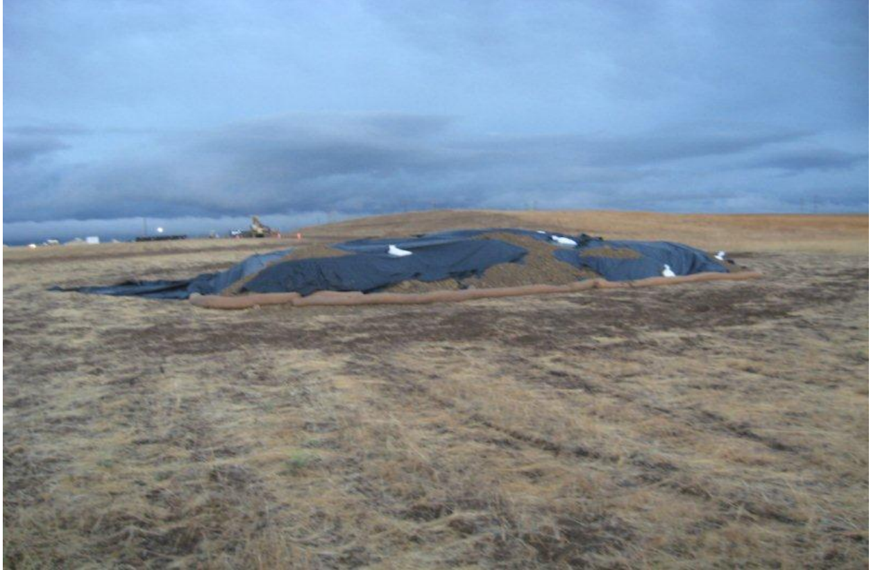
Photo 9, of alternate waterline spoil pile prior to forecast rain event, 9/24/14.
