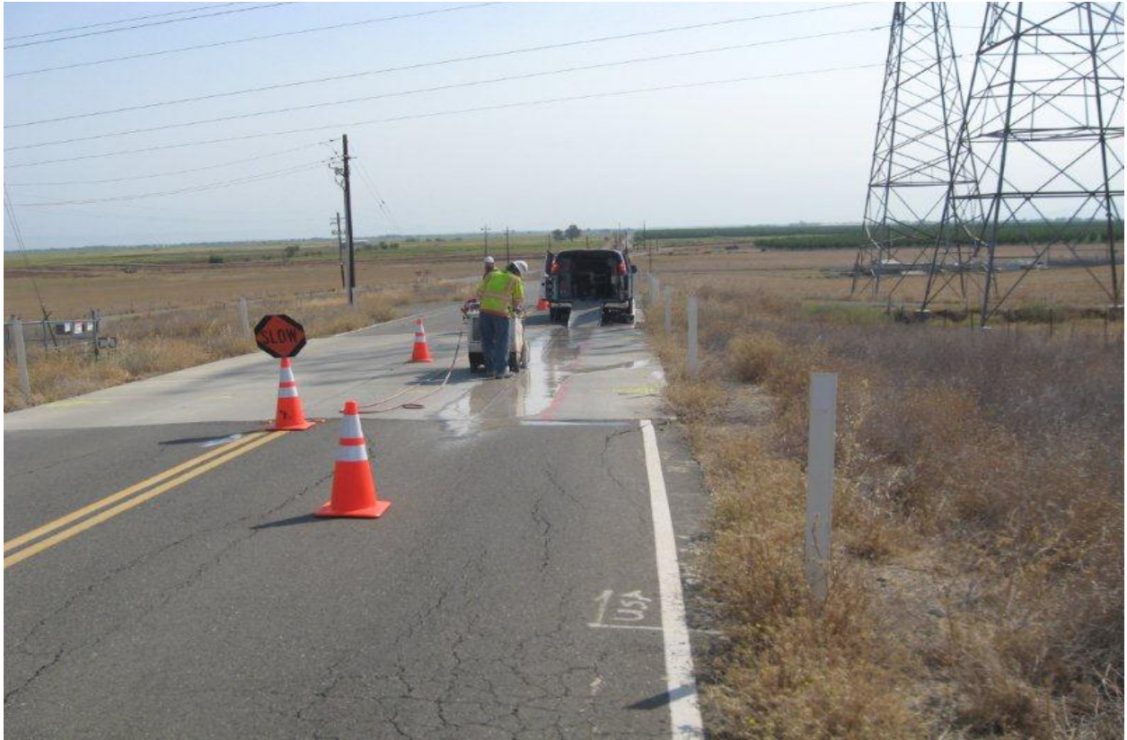
Photo 3, of saw cutting private entrance road to CGS facility for alternate waterline, 9/9/14.
