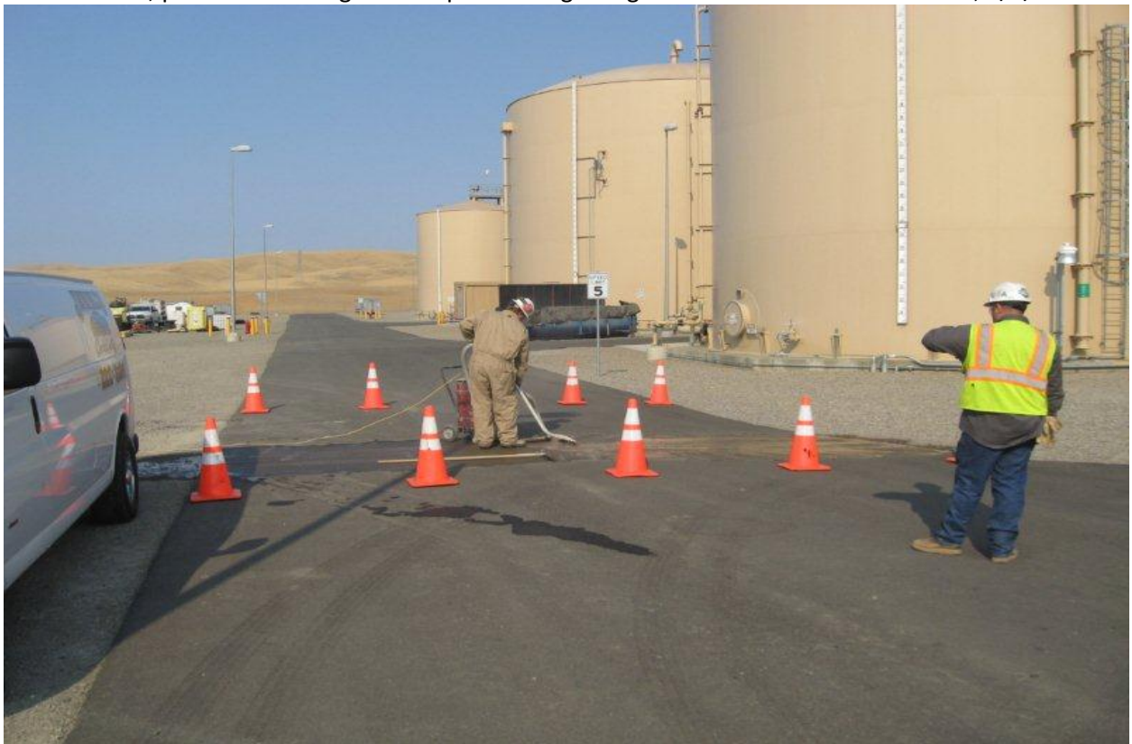
Photo 2, of saw cutting existing asphalt road within CGS facility for alternate waterline, 9/9/14.
