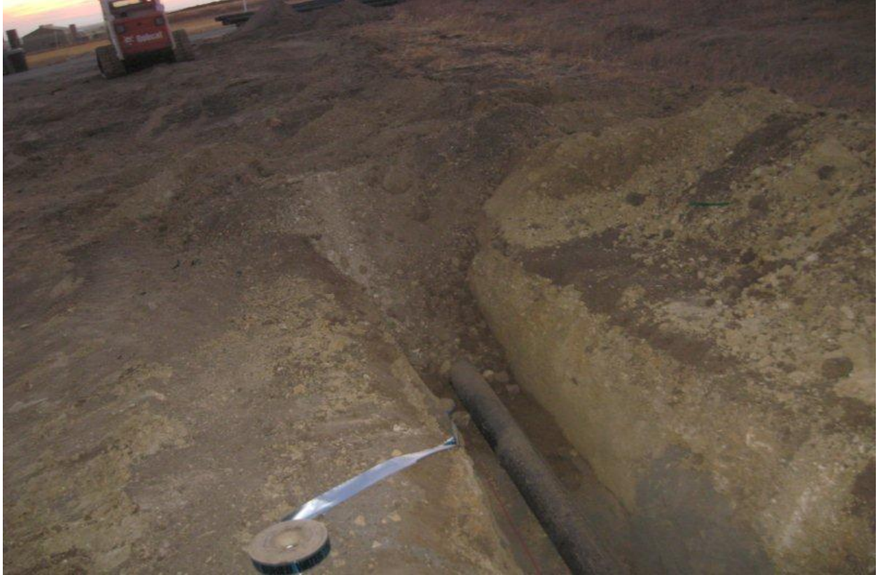
Photo 7, of typical pipe trench egress for potentially trapped wildlife, 9/23/14.
