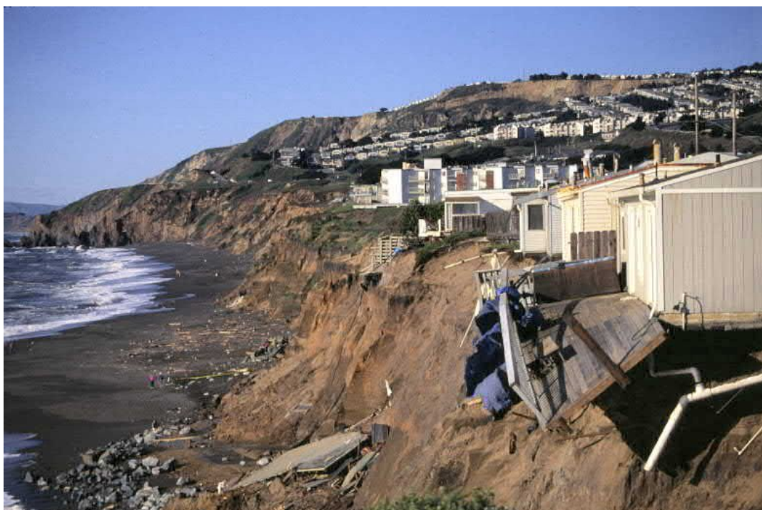
Figure D.4.6-28. Bluff Failure and Retreat During 1998 El Niño Storms, Pacifica, California (Photo by Kevin Coulton)
