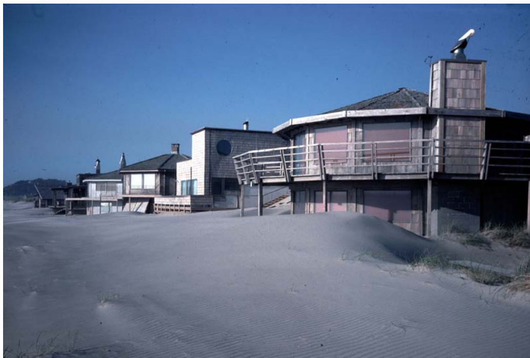
Figure D.4.7-4. Example of a Buried Coastal Structure that Could Affect Flood Hazard Zones and BFEs (top photo taken in 1978, bottom photo taken in 1988 – courtesy of Paul Komar)
