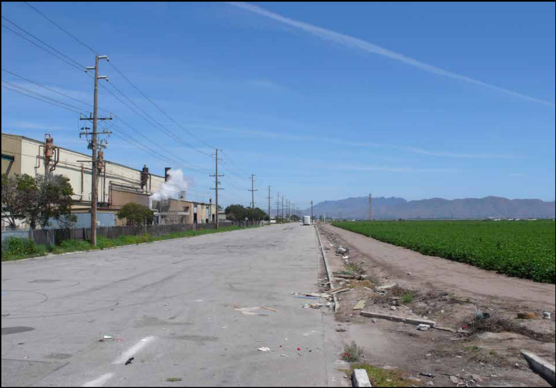
Puente Power Project - View East along E. McWane Boulevard from the Railroad Tracks West of Arcturus Avenue
