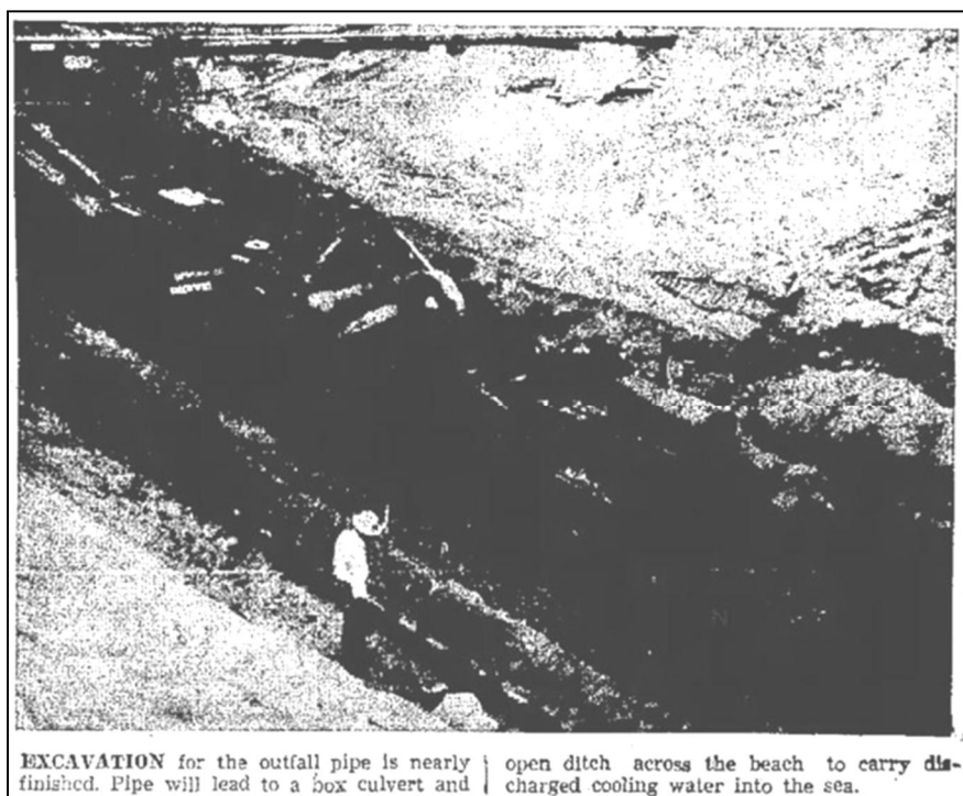
Oxnard Press-Courier, January 8, 1958. "Steely Skeleton Taking Shape on $75 Million Job."
