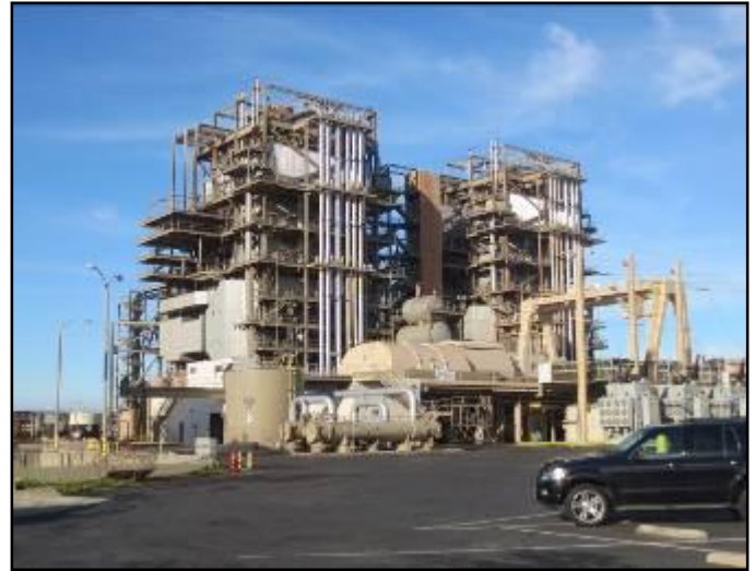
View of eastern and southern elevations facing northwest, displaying Units 1 and 2, de-aerator system.
