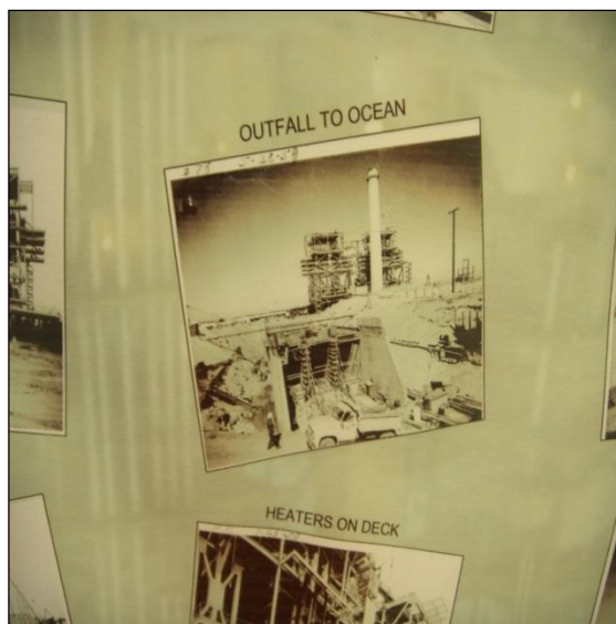
Display at MGS. Photograph of MGS Outfall construction in 1958.
