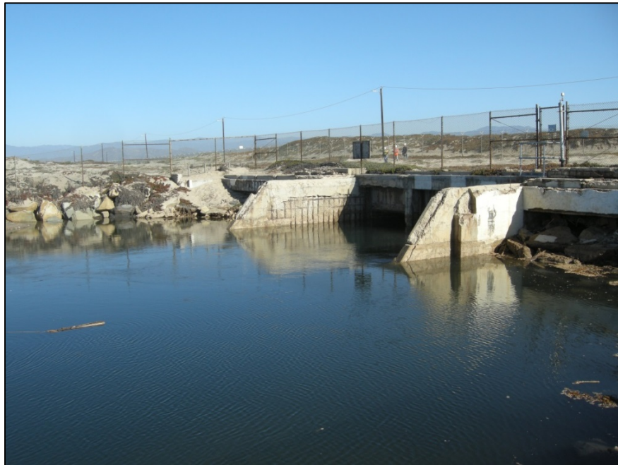
Figure 2. MGS Outfall, view to the northeast.
