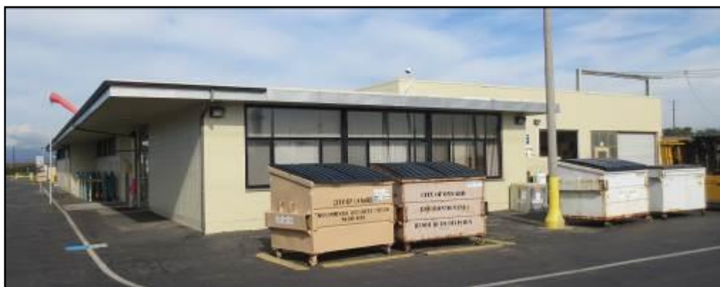
View of the maintenance building and garages, facing south.
