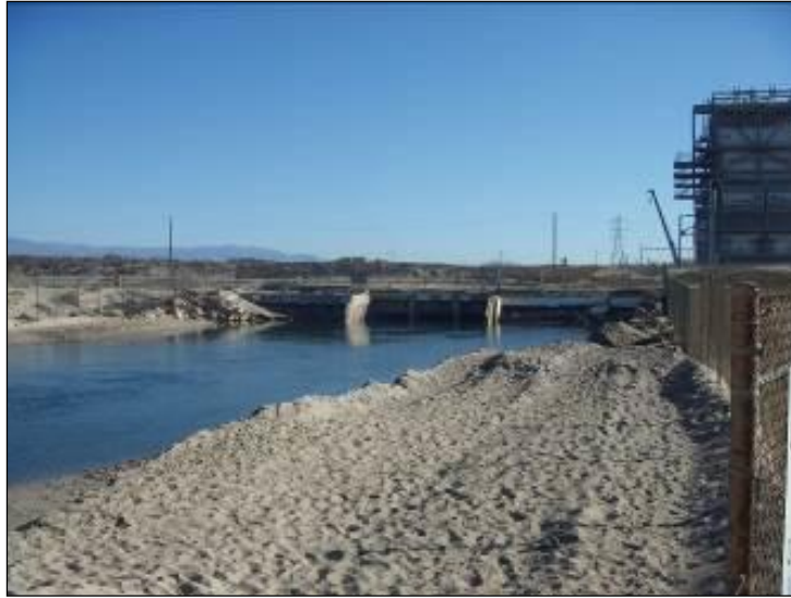
MGS Outfall; view facing northeast.
