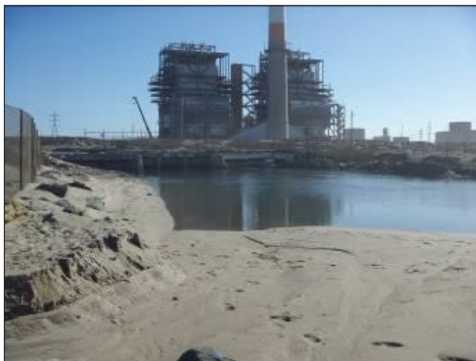
MGS Outfall; view facing southeast.
