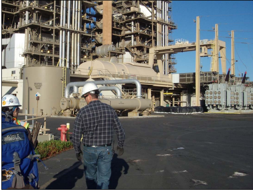
Figure 5. Proposed stormwater and wastewater utility area, view to the northwest
