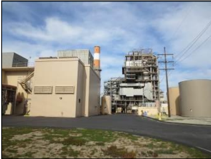
View of southern elevation of Unit 3 and storage tanks (foreground), with Units 1 and 2 and steam stack in the distance, facing north.
