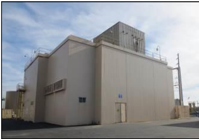
View of western and northern elevations of Unit 3, facing southeast.
