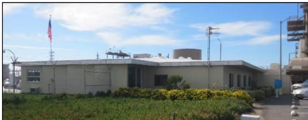
View of the administrative building, facing west.
