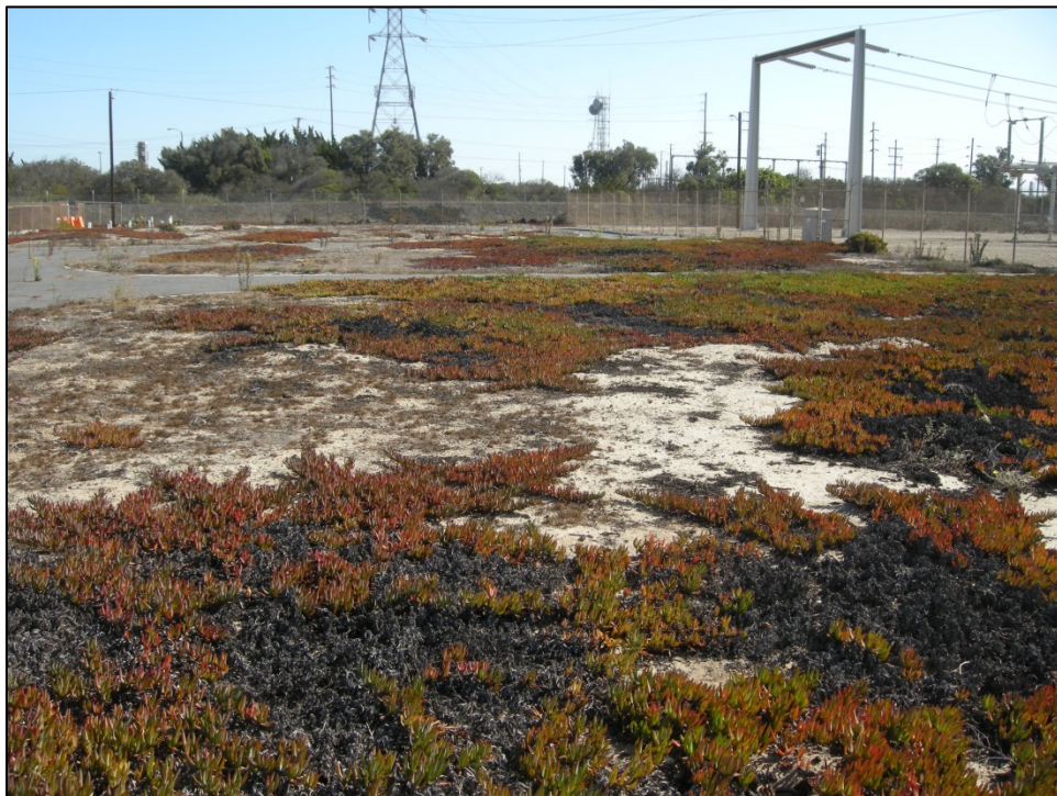
Figure 4. Proposed Take-Off Structure area south of Existing Construction Craft Parking, view to the east.
