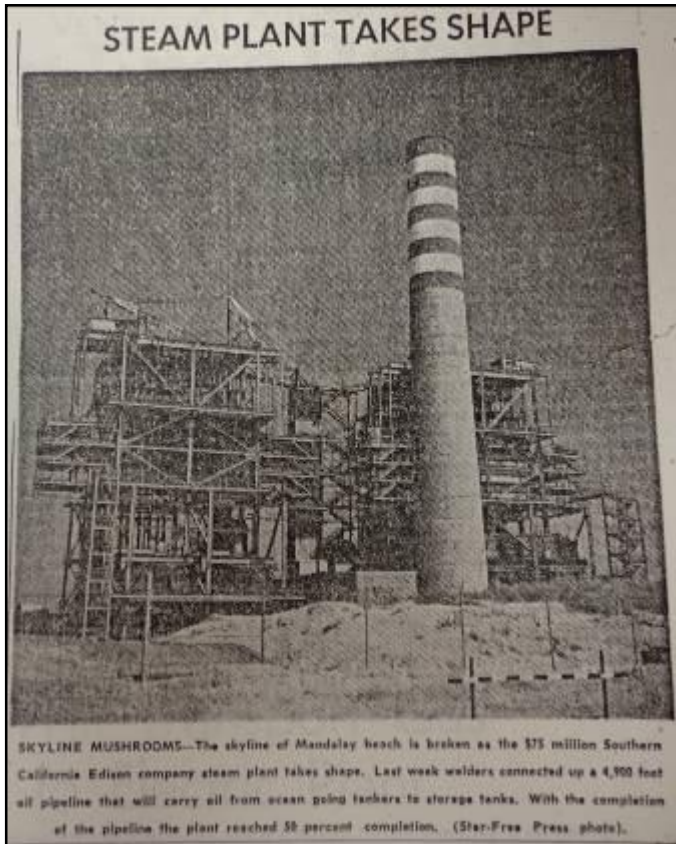
Photo from the Ventura Star Free Press, September 2, 1958. Caption discusses the construction of the MGS reaching 50 percent completion. (Source: Oxnard Public Library, Local History Room).
