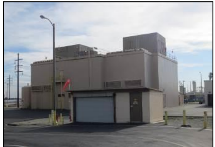
View of Unit 3 northern elevation and garage storage units, facing south.
