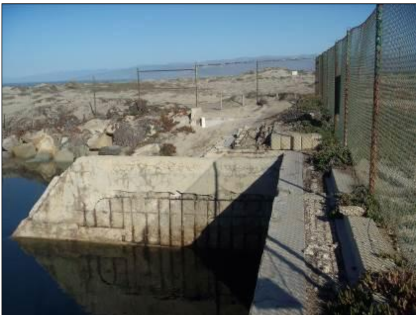
MGS Outfall platform; view facing north.
