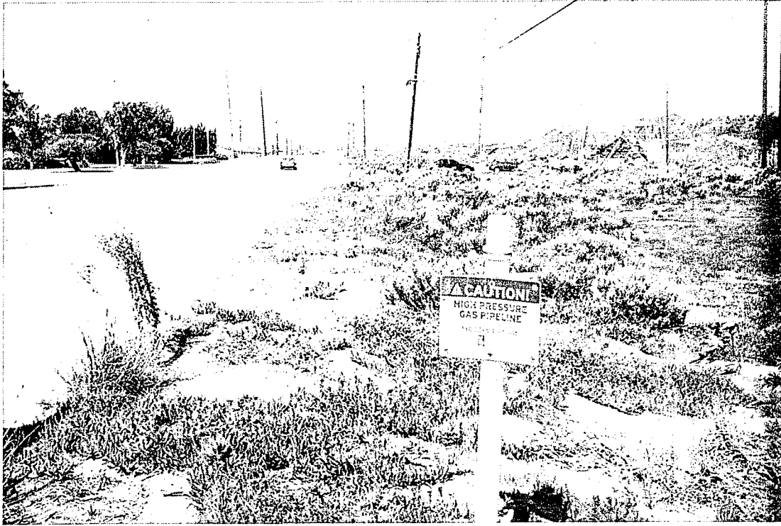
Photograph 5. This photograph depicts the location of the existing pipeline corridor. The proposed natural gas pipeline route is to be installed between the existing pipeline corridor and Harbor Boulevard. Photograph taken on October 13, 2008.
