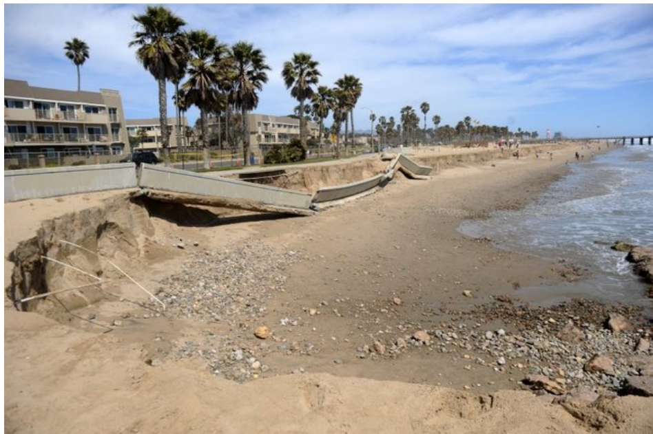
Figure 7. Erosion at City of Port Hueneme following a multi-year gap in dredging (photo courtesy Ventura County Star)
