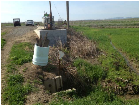
Photo 27, looking south at freshwater marsh along edge of irrigated winter wheat field. Note culvert box which leads to drainage canal in photo 29.
