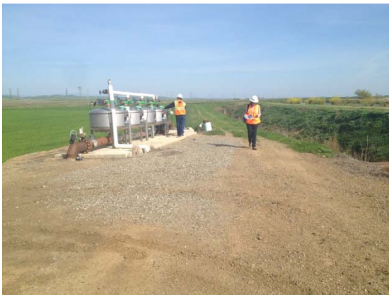
Photo 21, looking north at proposed water intake location adjacent to property owner's water intake and filtration station.
