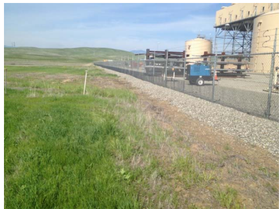
Photo 6, looking west at primary waterline alignment on south side of CGS.
