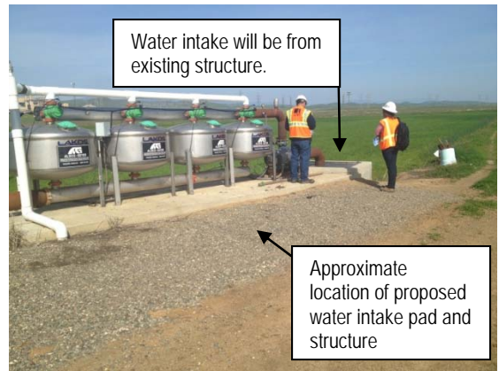
Photo 22, looking northwest at water intake.
