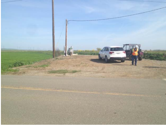
Photo 19, Looking north at proposed water intake pad adjacent to property owner's intake and filtration station.
