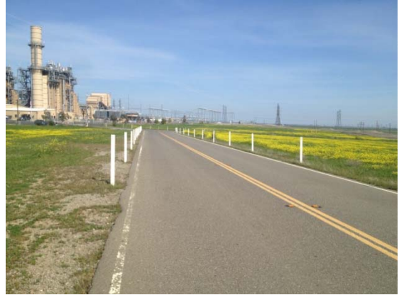
Photo 8, looking north at waterline alignment within edge of right paved road.
