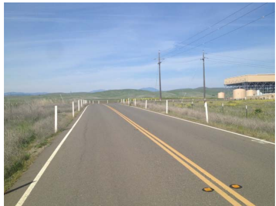
Photo 10, looking west toward curve in road as seen in Photo 9.
