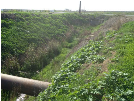
Photo 29, looking south at drainage canal at east side of water intake pad. Pipe is existing water intake line for property owner out of the Glenn-Colusa Canal.
