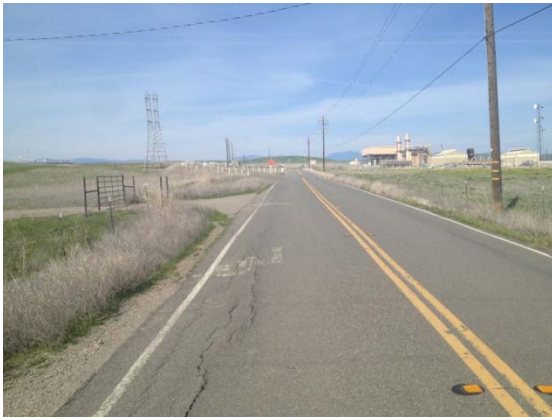
Photo 15, looking west at waterline route through disturbed grasslands.
