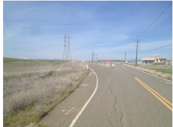
Photo 14, looking west where road splits near Delevan Compressor Station.
