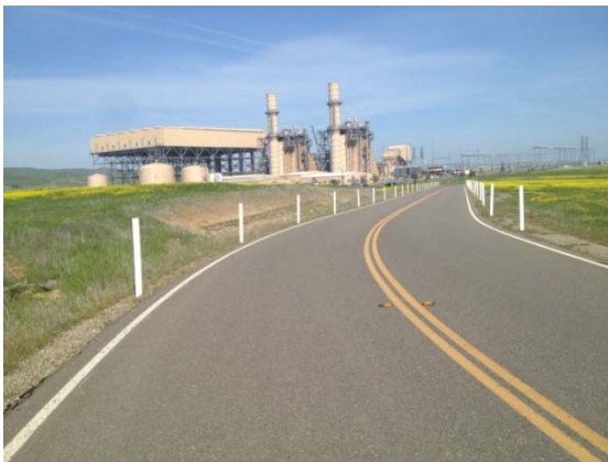
Photo 9, looking north at waterline route.
