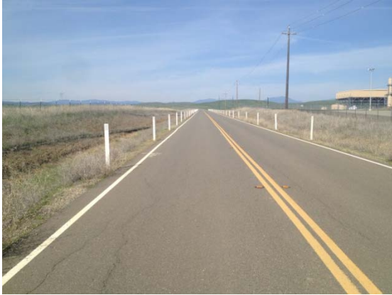
Photo 13, looking west at waterline alignment through disturbed California annual grasslands adjacent to Delevan Compressor Station.
