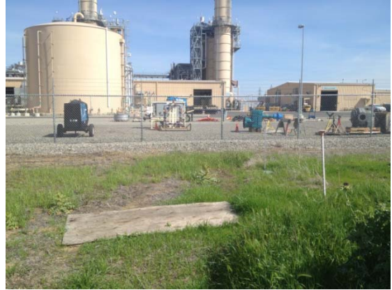
Photo 2, looking north where waterline will enter CGS into building in background.
