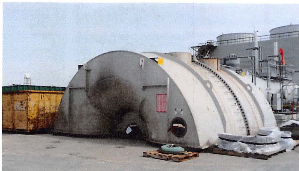
Figure 3. Steam Turbine Housing that has been removed
