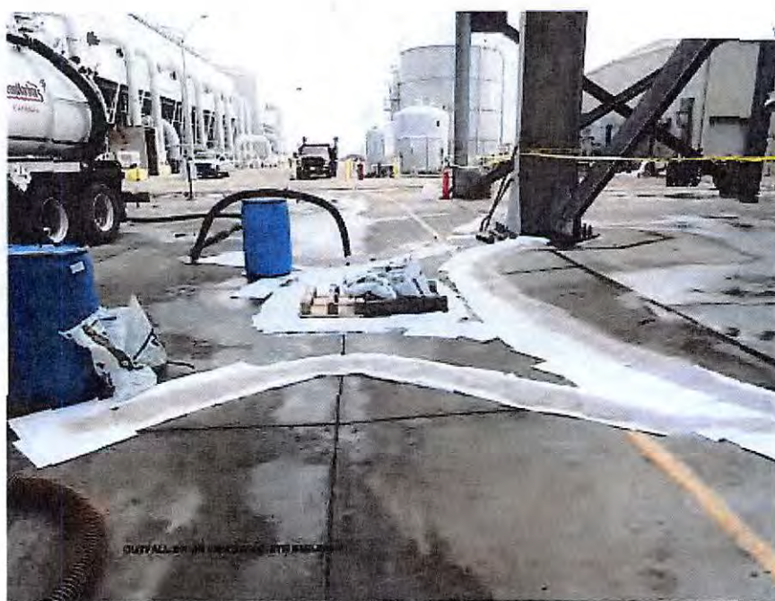
Figure 3. A Blocked Outfall Drain On West Side Of The Steam Generator Turbine Enclosure During Clean-up
