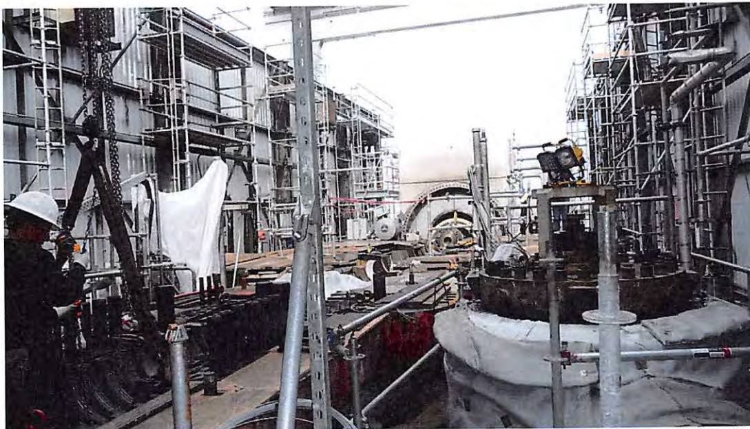
Figure 9. Steam Turbine Building with roof and steam turbine removed
