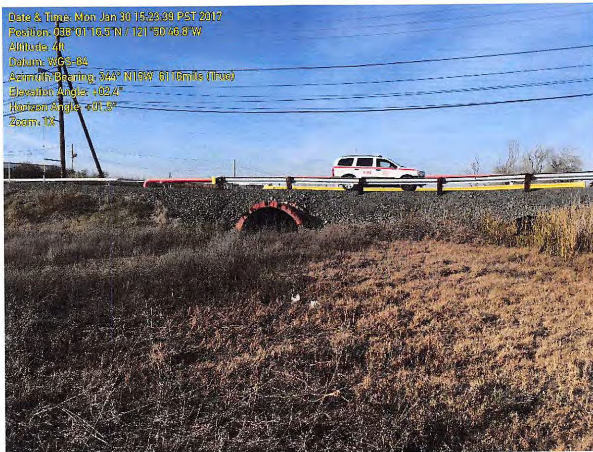
Photo 6. View to the north from Dowest Slough showing large culverts beneath East 5 th Street. The culvert to the east is partially hidden behind tule and cattail that border the low flow channel. At the time of this photograph, flow to the south was observed through the east culvert.
