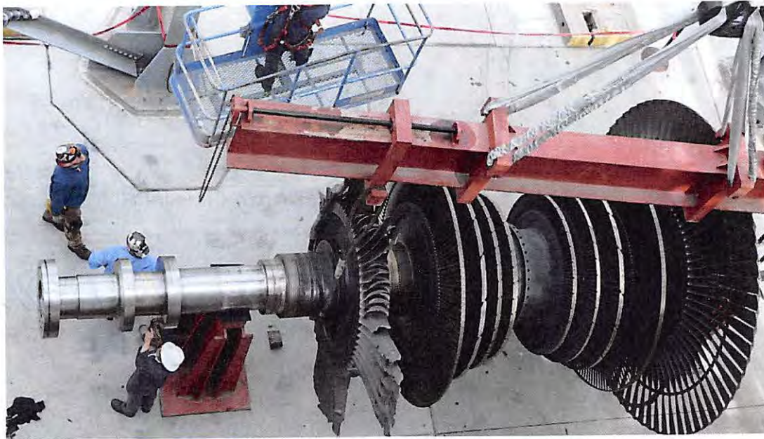
Figure 8. Steam Turbine Rotor removed for repair showing severely damaged blades
