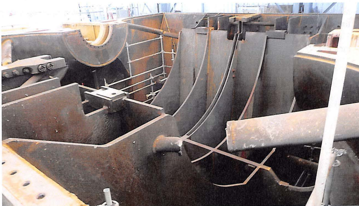
Photograph 2. View of Low Pressure Turbine Area Downward Steam Entrance to Condenser
