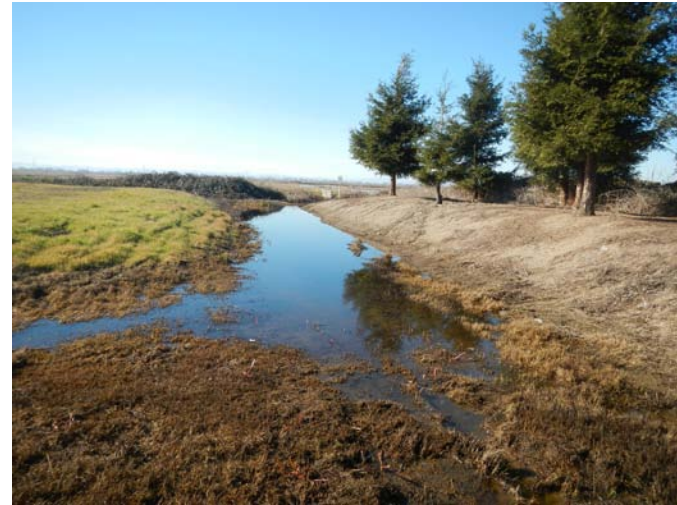
G-22. SEC Wetland Delineation: View west of ponding due to overflow from drainage ditch at DP Outfall B. January 18, 2013.
