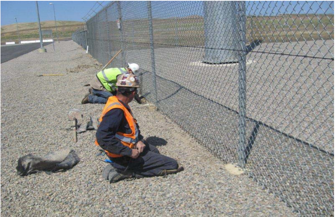
Photo 10, of CGS employees repairing snake fencing near CGS switch yard, 5/2/13.
