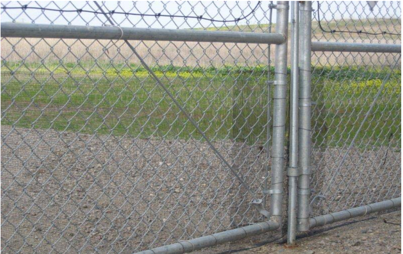
Photo 2, snake fencing applied to outer perimeter fencing around CGS site, 3/4/13.
